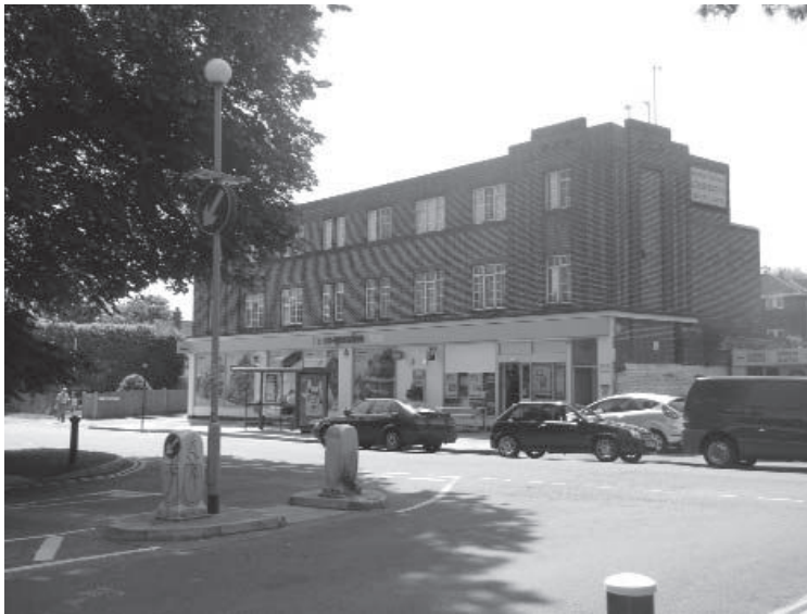
figure 6 - Junction with Ladies Mile Road
